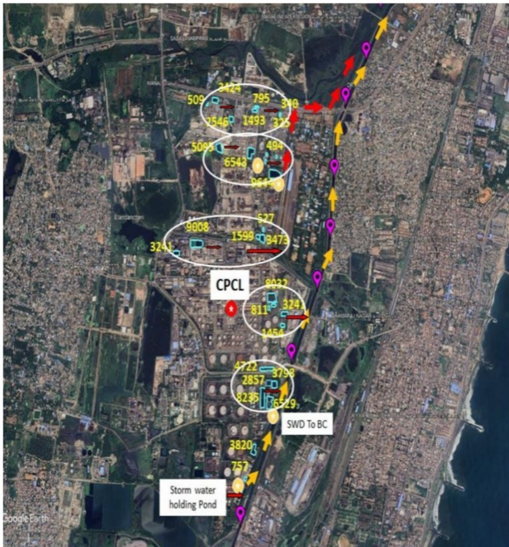
Figure 34: Open tank locations and area in sq.m.
