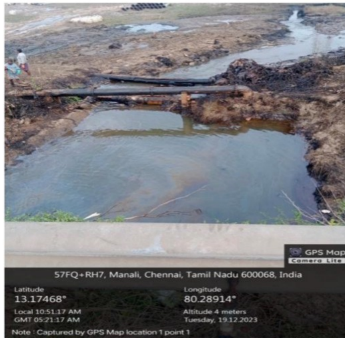
Figure 12: Close up view of Zone 1
