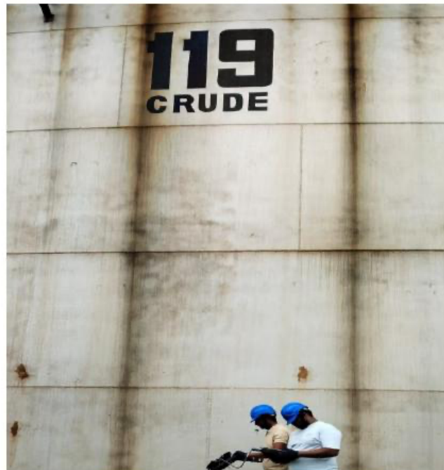
Figure 13 shows site photograph taken during the GPR scanning process for tank 119.
